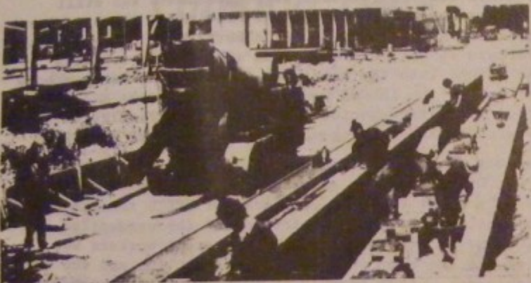
The £20m. Ferenka Plant under construction at Annacotty, Co. Limerick
